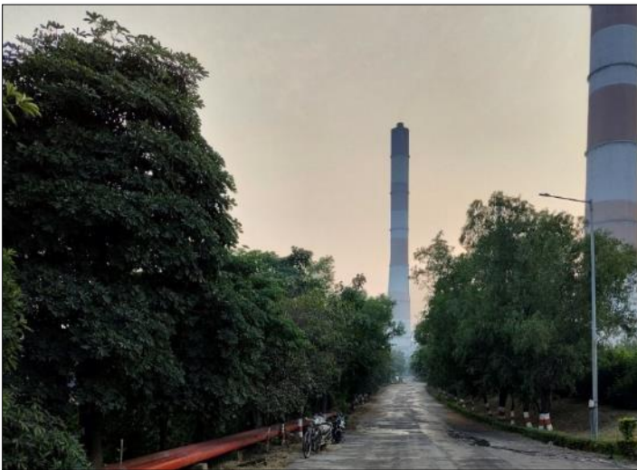
DM Plant Road
