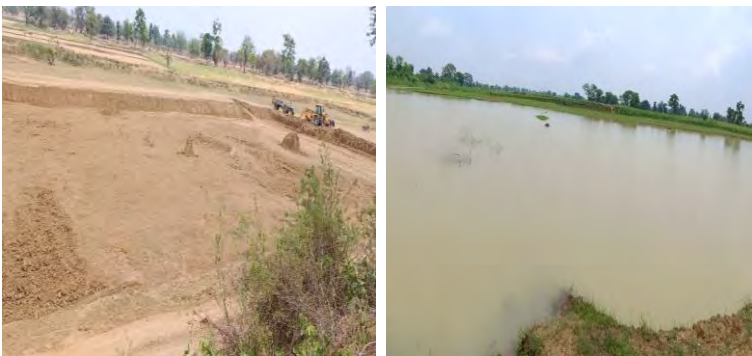
Pond Deepening – Garada Village
