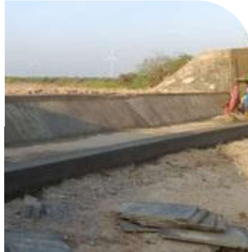
Renovation of Check dam at Pavadiyara village - 300 people benefited
