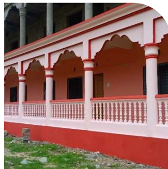
Renovation of High School at Zaarapa – 2200+ Benefited
