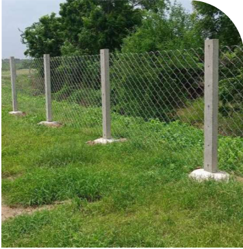
Construction of chain-link fencing at Mangra village – 300 people benefited
