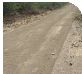
Renovation of approach road, Zarpara – benefiting 400 villagers
