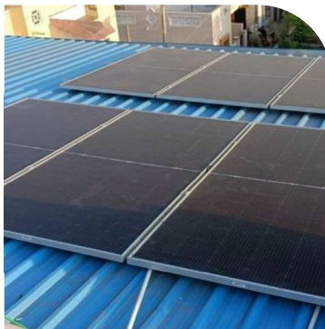
Supply & installation of Solar panel (3.25 KV) at CGP, Mundra – benefiting 1200 people
