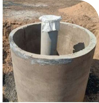
Construction of 21 Borewell Recharge in Nagmati River - 150+ farmer benefited
