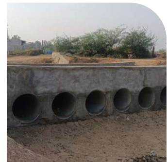
Construction of Pipe Culvert – 400+ Benefited
