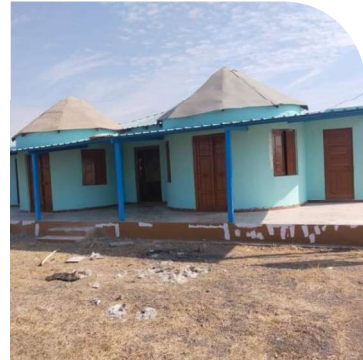
Renovation of Balwadi at Juna bandar & Luni bandar
