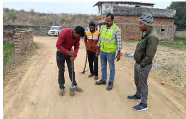
6 KM Approach Road Repairing in Core Village
