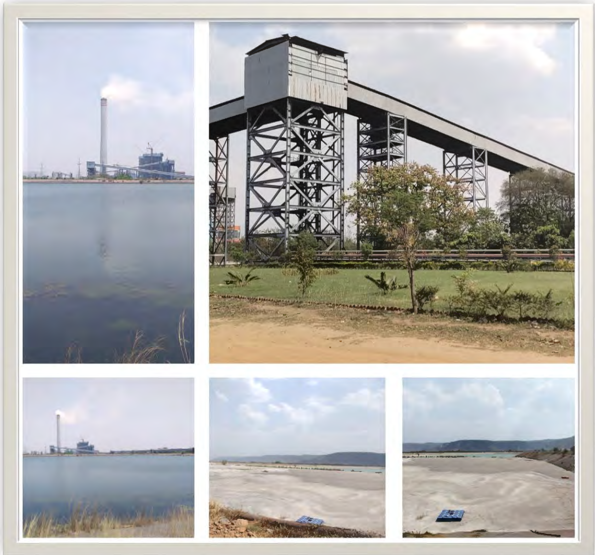
FIGURE 1.3: VIEW OF MAHAN TPP AT SINGRAULI MADHYA PRADESH
