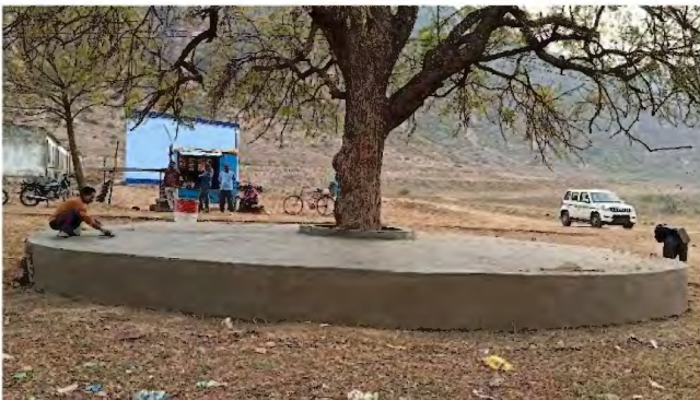
Seating Chabutra construction at Nagwa.
