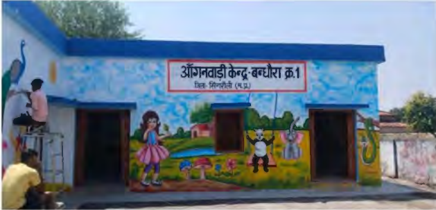
Renovation of Anganwadi, Bandhaura
