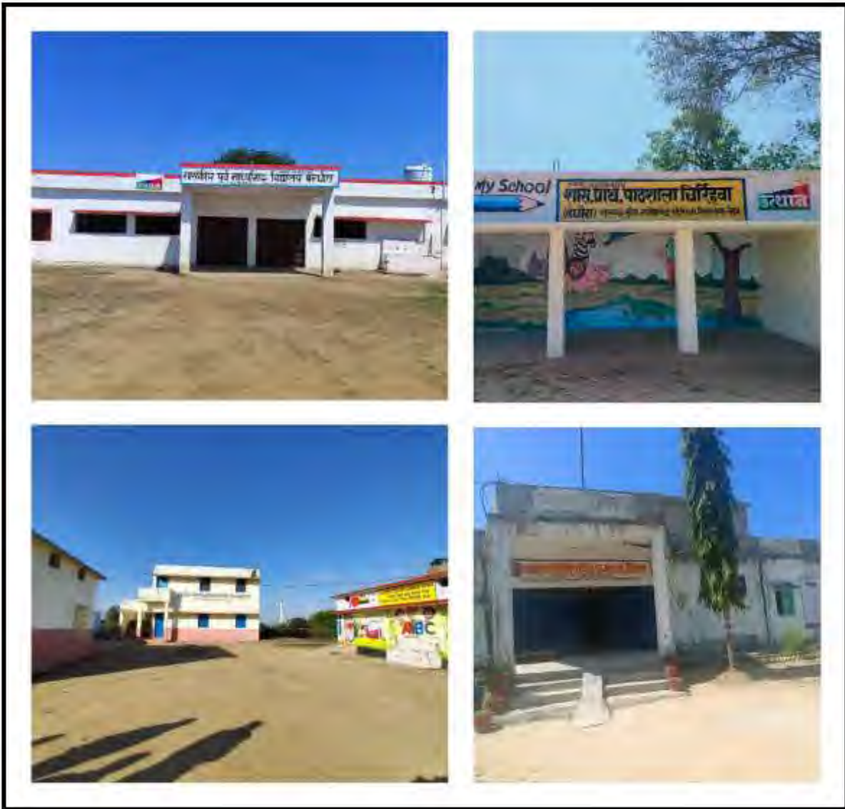
FIGURE 3.4: IDENTIFICATION OF PUBLIC LAND FOR GREEN BELT DEVELOPMENT AT SELECTED LOCATIONS AROUND MAHAN TPP
