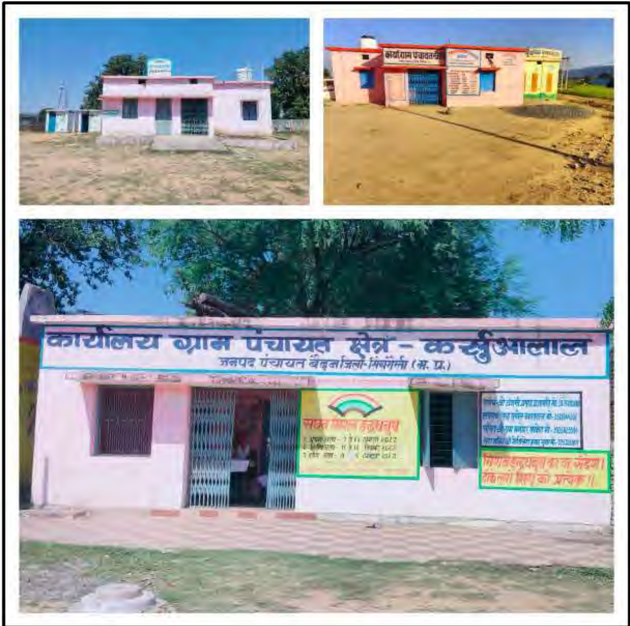
FIGURE 3.5: IDENTIFICATION OF PUBLIC LAND FOR GREEN BELT DEVELOPMENT AT SELECTED LOCATIONS AROUND MAHAN TPP
