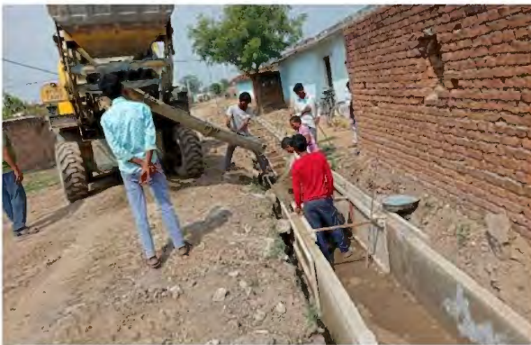
1.1 KM Drain Construction in R&R Colony
