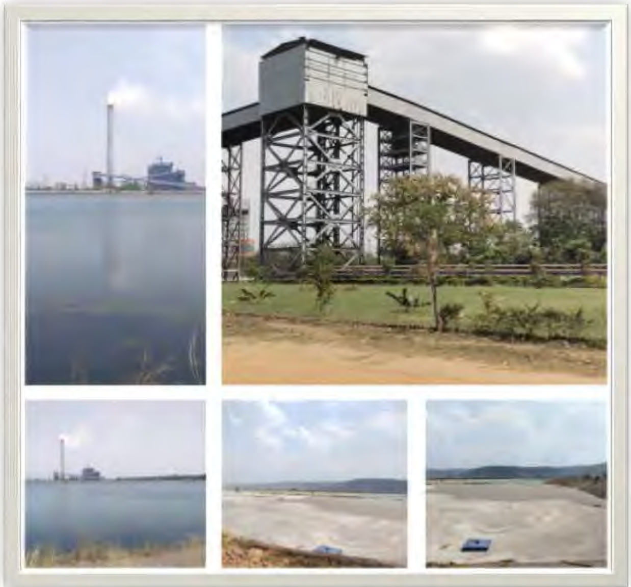
FIGURE 1.4: VIEW OF MAHAN TPP AT SINGRAULI MADHYA PRADESH
