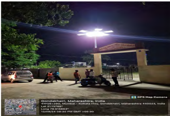
Installation of High Mast Solar Light
